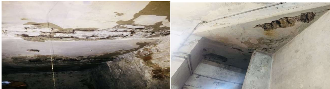
Fig.4 Spalling & Corrosion of reinforcement in structural element
