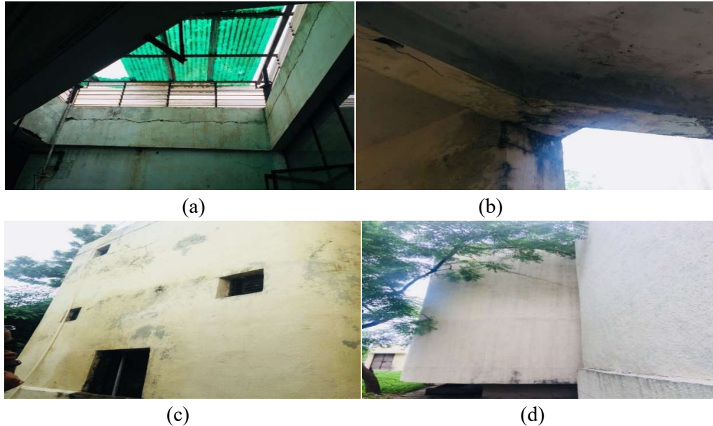
Fig.3 Different Cracks (a) bonding crack (b) longitudinal crack (c) shrinkage crack (d) diagonal crack
