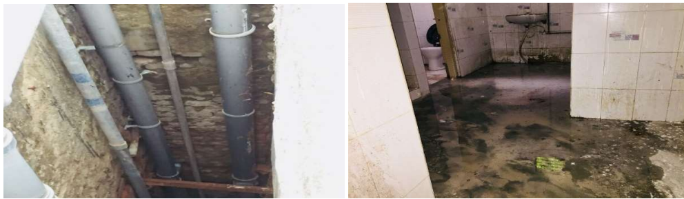
Fig. 6 Peeling of paints and dampness effects
